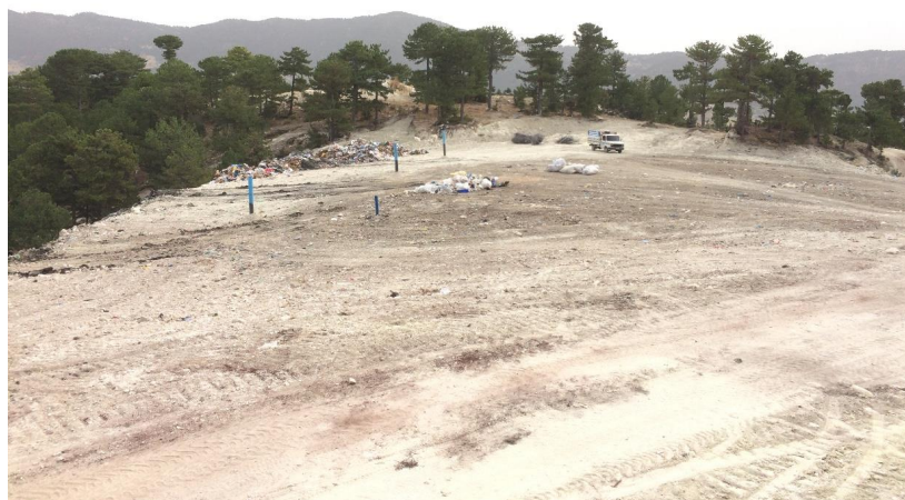
b) Cameli, Denizli open dump after rehabilitation
